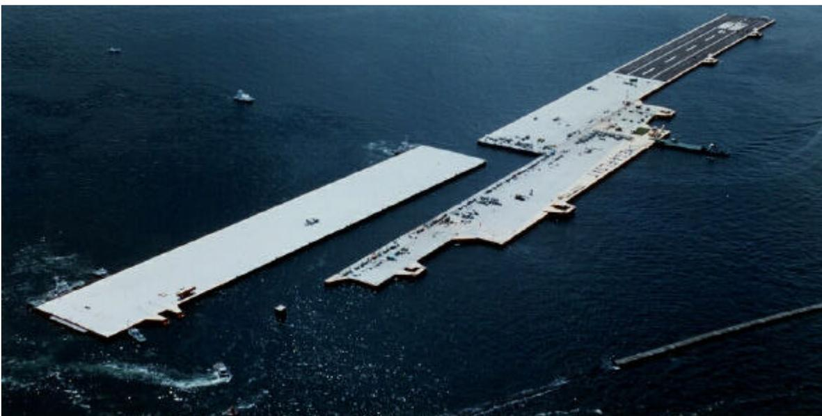
FIG-1 :View of the experimental model in Phase-1 (joining of unit on sea)
