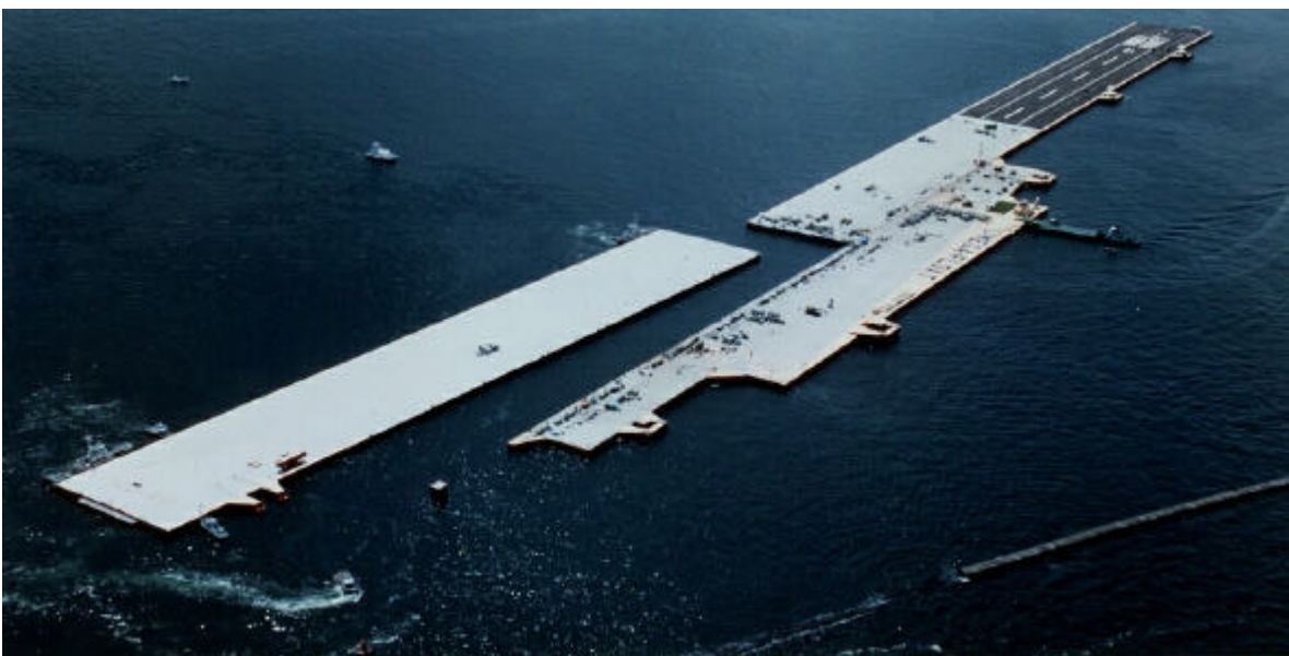
FIG-1 :View of the experimental model in Phase-1 (joining of unit on sea)
